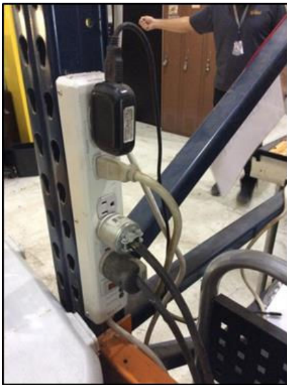
(Power strips permanently mounted / daisy chained)
