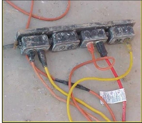
(Electrical outlet boxes used for temporary power supply)
