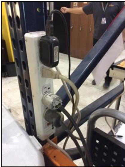
(Power strips permanently mounted / daisy chained)
