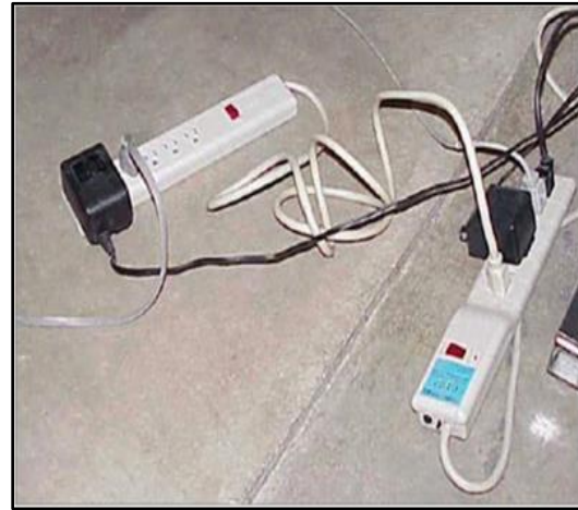
(Power strips permanently mounted / daisy chained)
