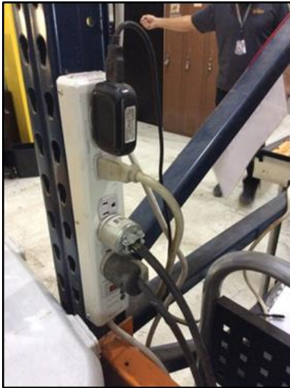
(Power strips permanently mounted / daisy chained)
