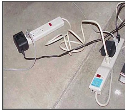
(Power strips permanently mounted / daisy chained)
